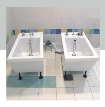
This unit is composed of two vats of rectangular form. Each vat includes a mitigated water feeding with nozzle, filling tap and overflow. A thermostatic mixer is localised on one of the 2 vats and ensures the control of water temperature.
